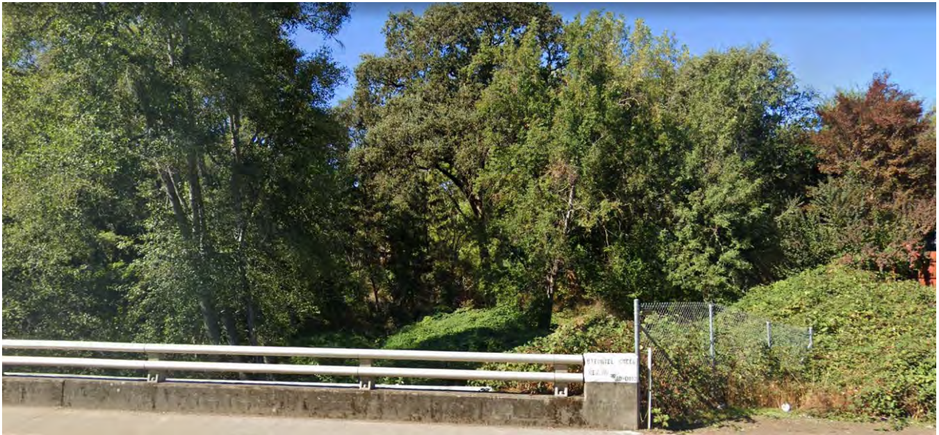
Figure 3.1b: View of Baechtel Creek from Highway 20/South Main Street Looking West
